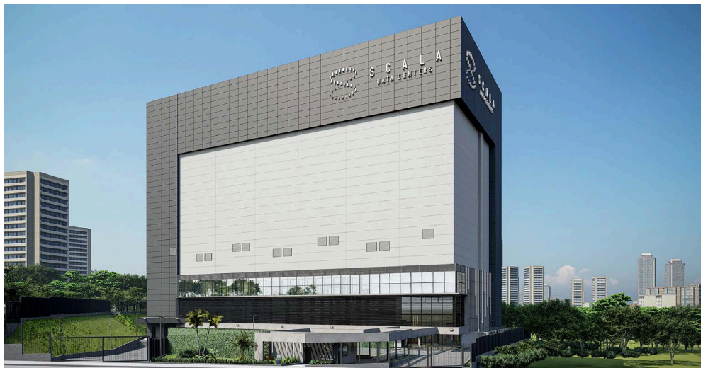
Largest vertical data center in the region (Scala)
